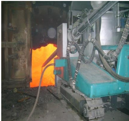
Hot Repair Spray of Converter
